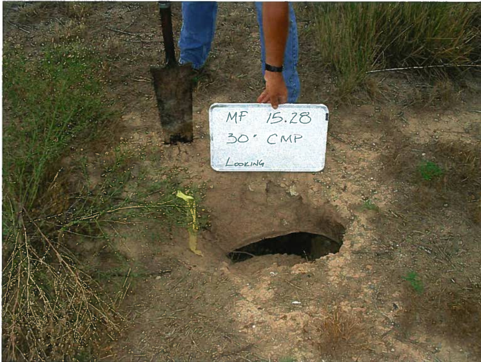
Mile Post 15.28 30" CSP South End
