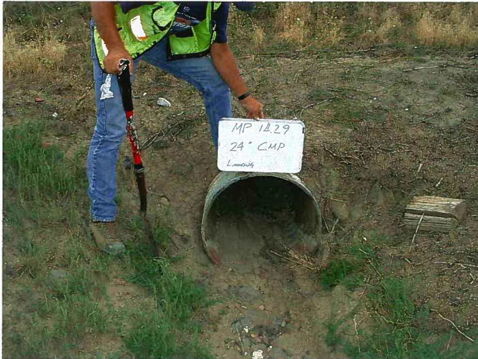
Mile Post 14.29 24" CSP North End
