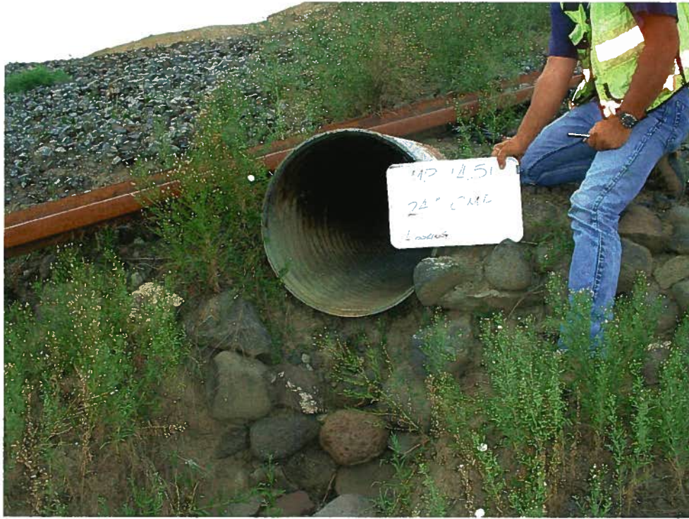
Mile Post 14.51 24" CSP South End
