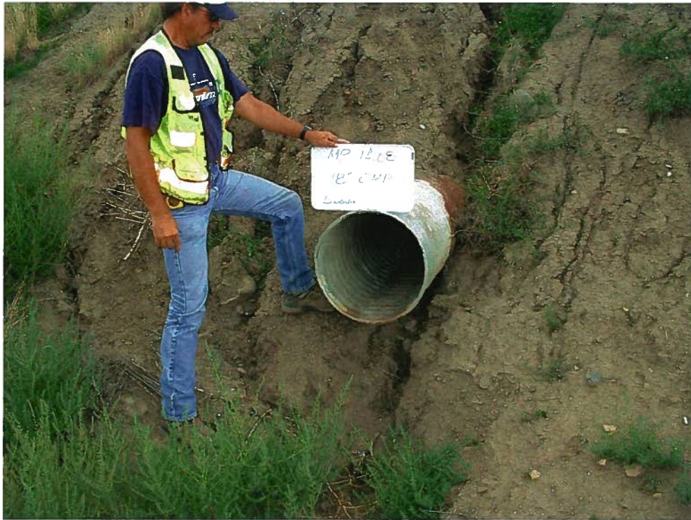
Mile Post 14.08 18" CSP South End
