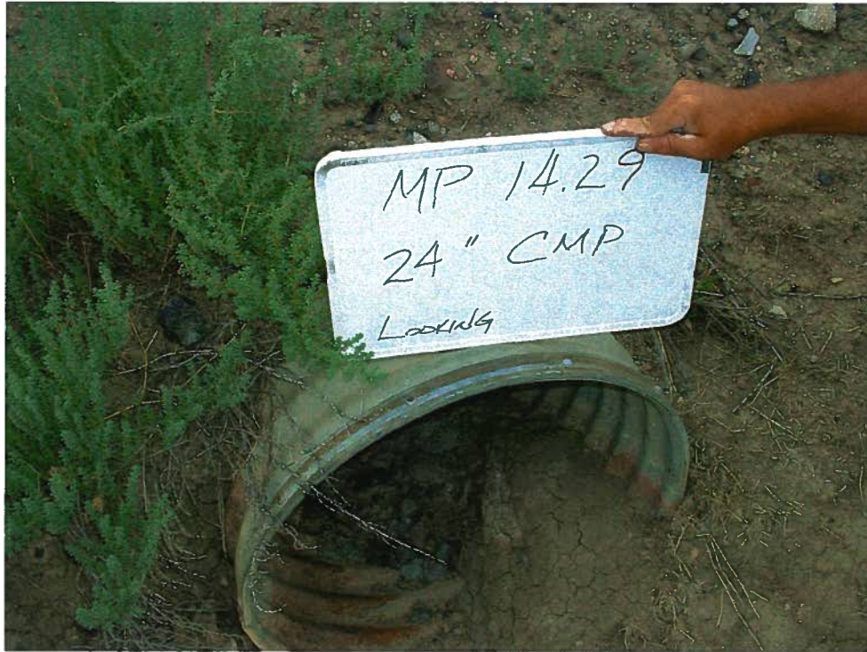
Mile Post 14.29 24" CSP South End
