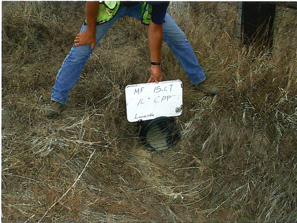
Mile Post 15.07 10" CPP South End
