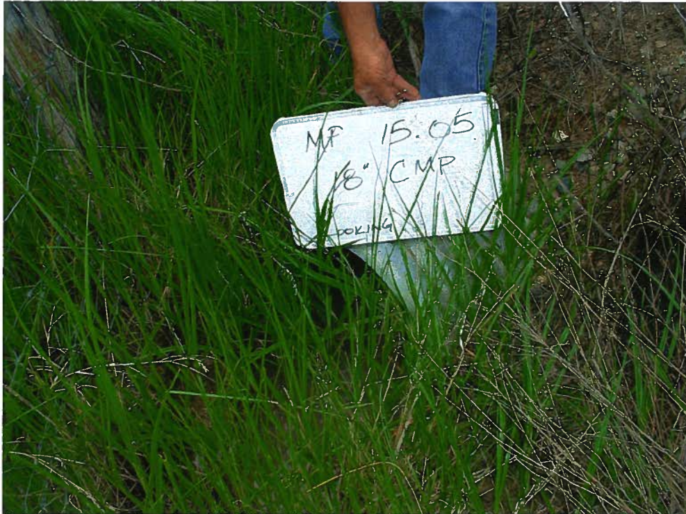
Mile Post 15.05 18" CSP East End
