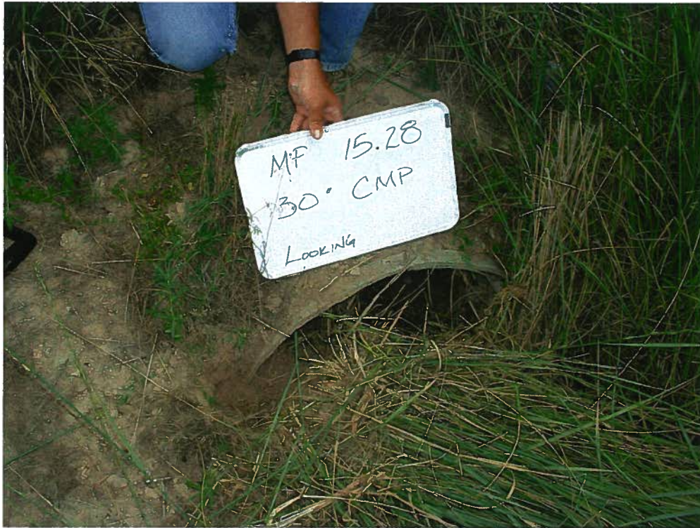
Mile Post 15.28 30" CSP North End
