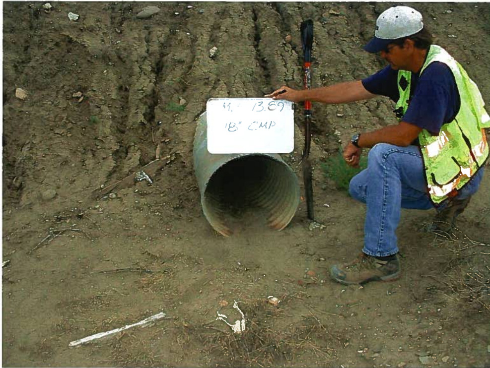
Mile Post 13.89 18" CSP South End
