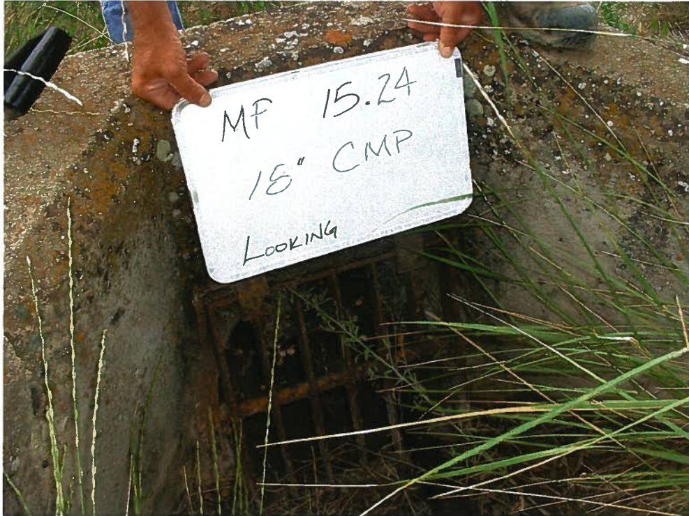
Mile Post 15.24 18" CSP North End
