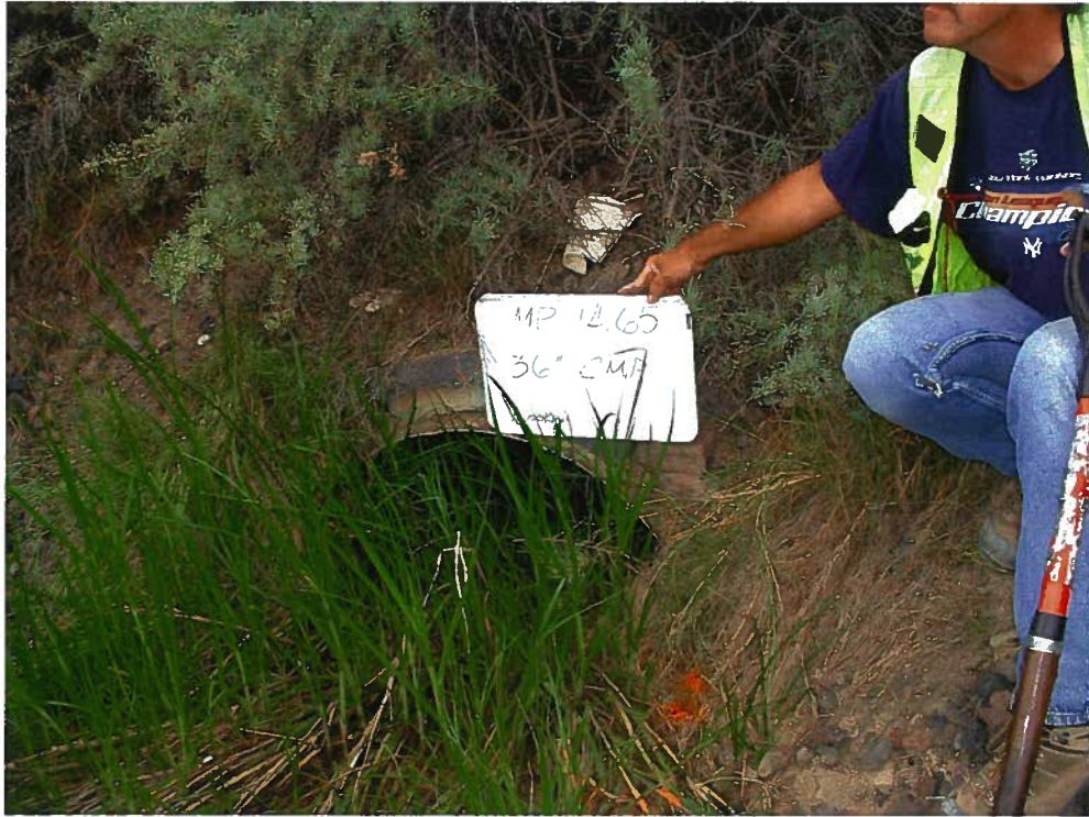
Mile Post 14.65 36" CSP South End
