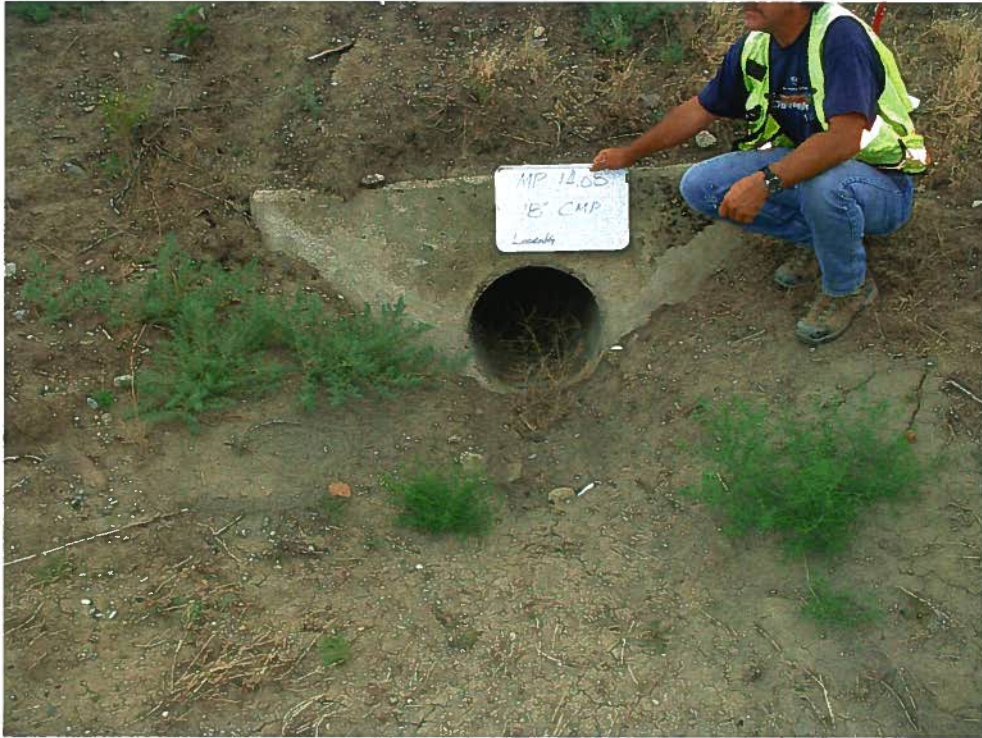
Mile Post 14.08 18" CSP North End
