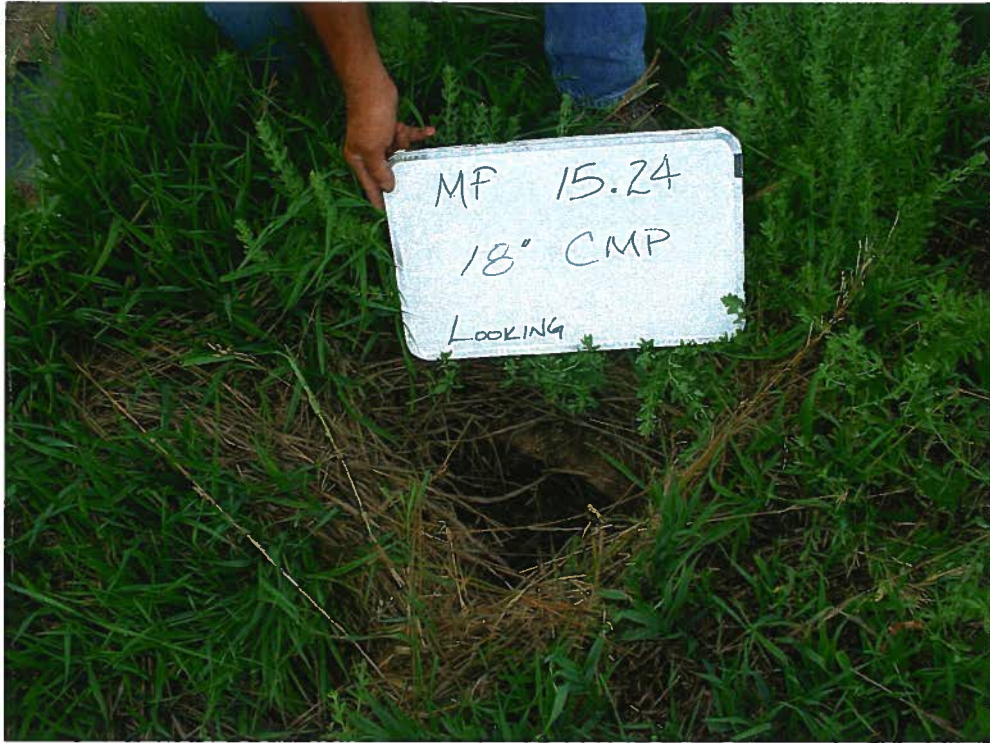
Mile Post 15.24 18" CSP South End
