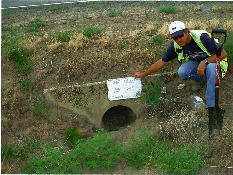
Mile Post 14.00 18" CSP North End
