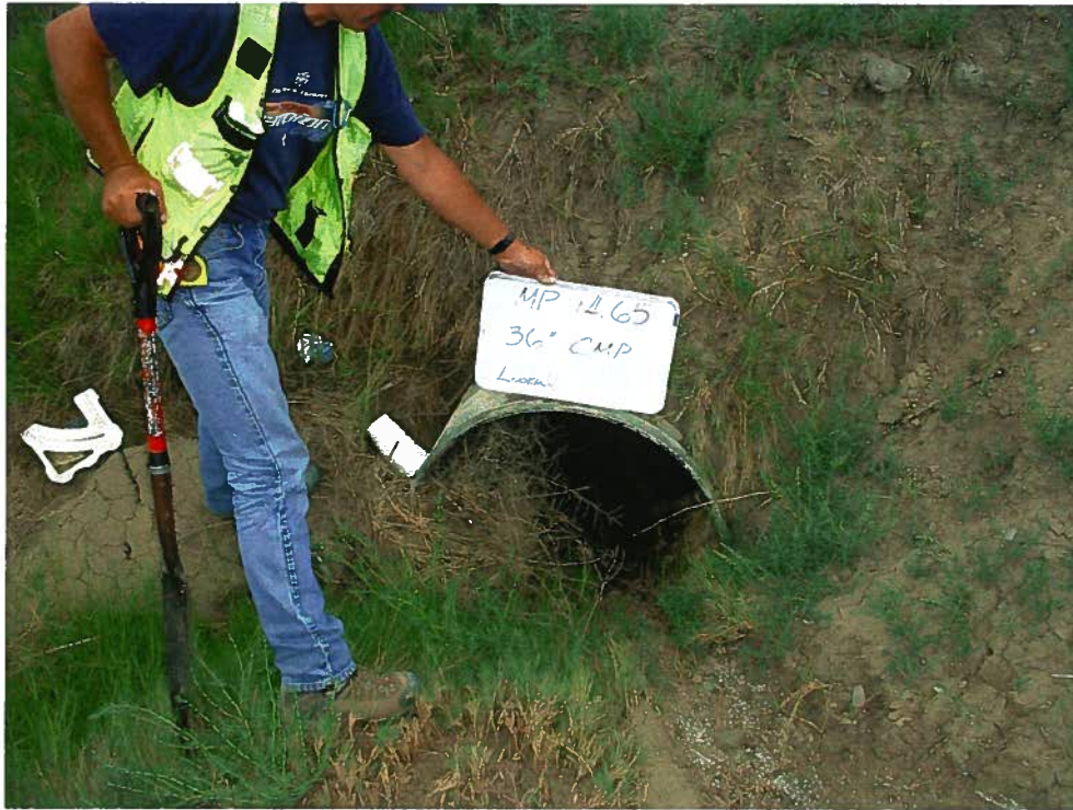
Mile Post 14.65 36" CSP North End
