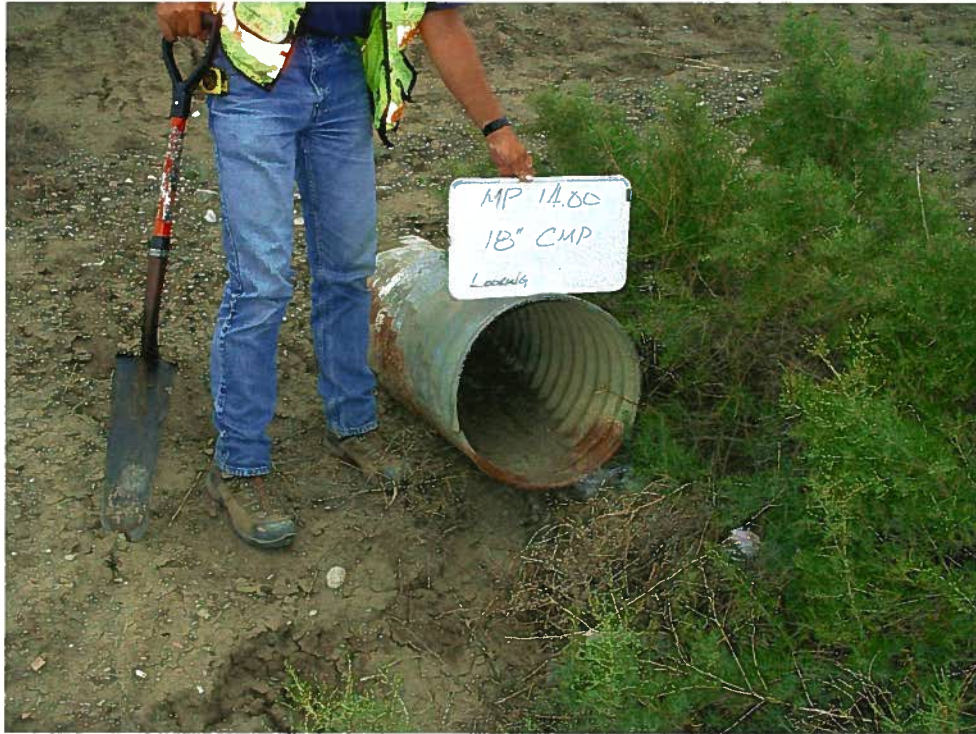
Mile Post 14.00 18" CSP South End
