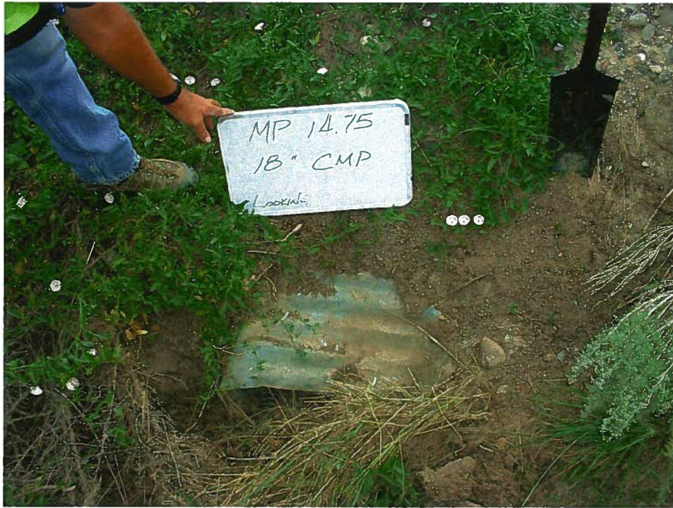
Mile Post 14.75 18" CSP East End
