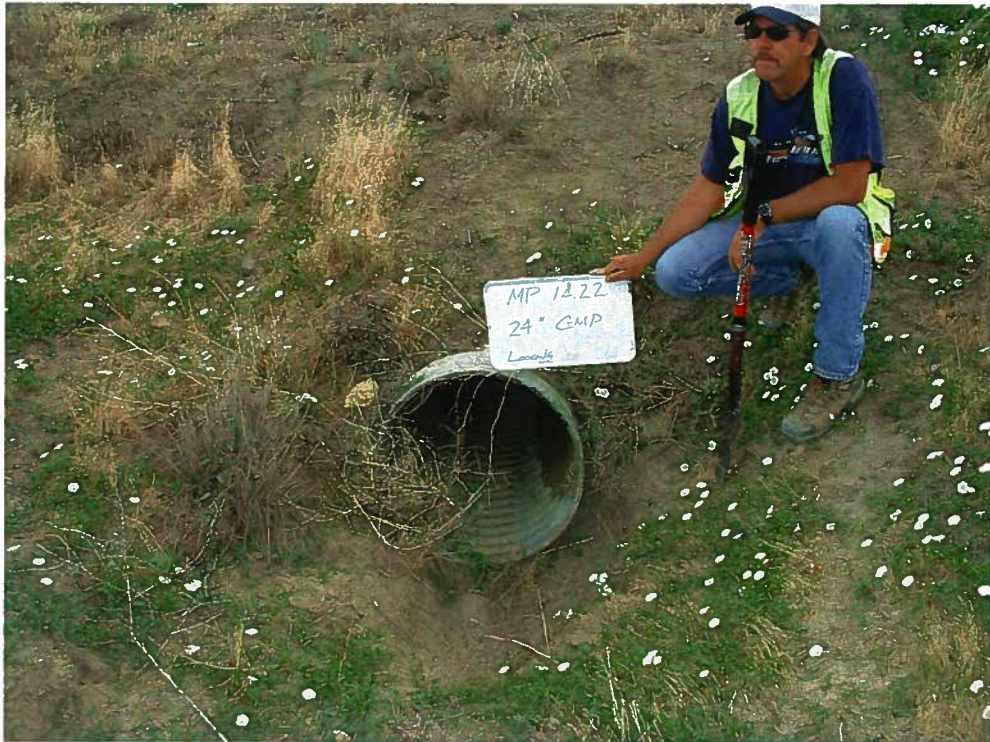
Mile Post 14.22 24" CSP North End
