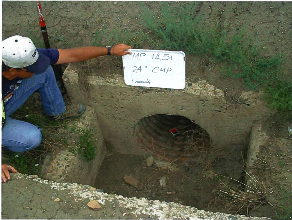
Mile Post 14.51 24" CSP North End
