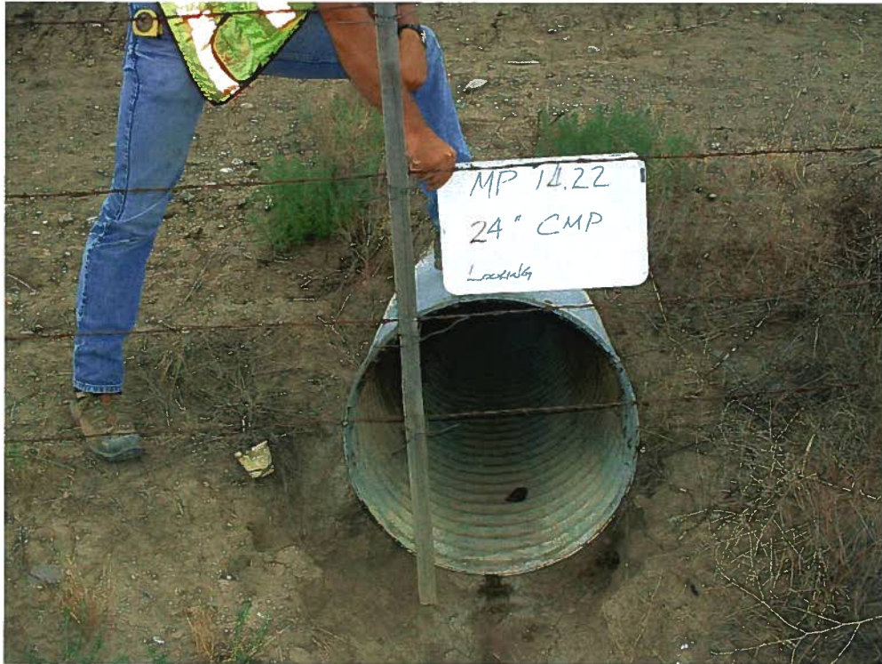
Mile Post 14.22 24" CSP South End
